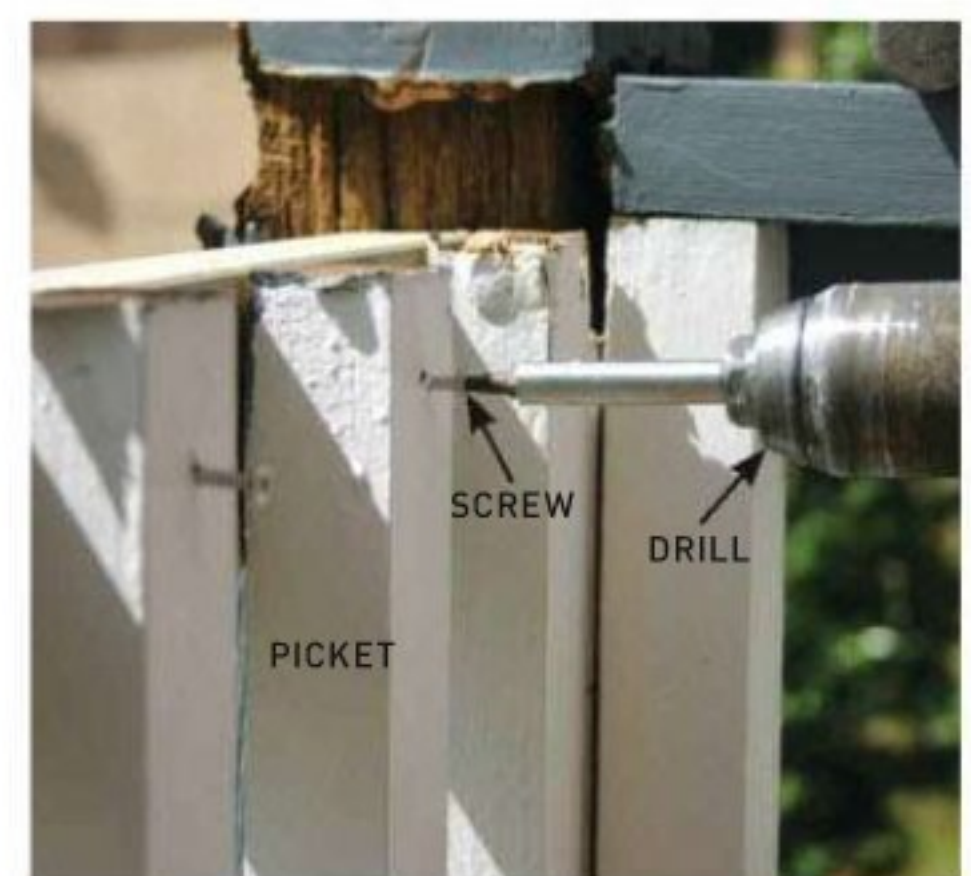
After The deck balustrade will last much longer after the repairs.
