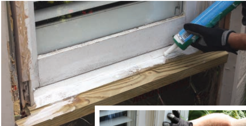
I fastened the sill with a combination of shims, decking screws and silicized adhesive sealant.
