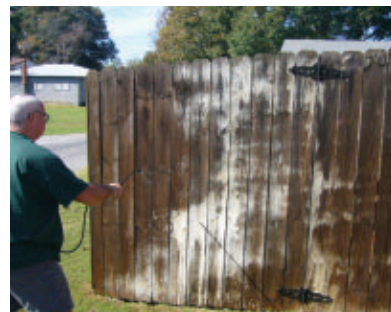
The cleaning agent was applied with a sprayer to remove mold and mildew and open the wood-grain to better absorb the stain.
