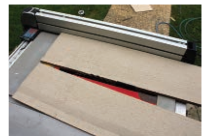
I had to rip the final siding panel to fit beneath the window.
