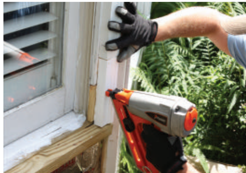
I fastened the sill with a combination of shims, decking screws and silicized adhesive sealant.
