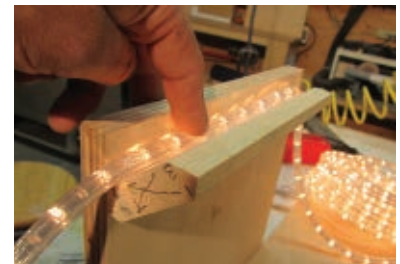
The lighting should remain hidden in the channel behind the molding to provide soft, ambient lighting.
