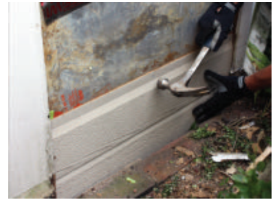
Siding installation begins at the bottom.
