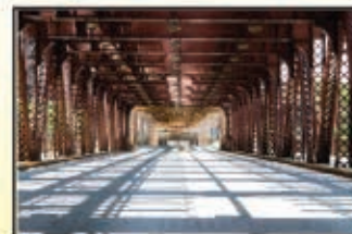
Heavy metal paint bridge restoration
