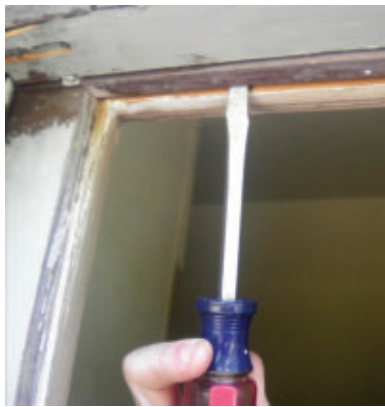
The top edge of the pane includes a groove, which the top of the glass pane slips into.
