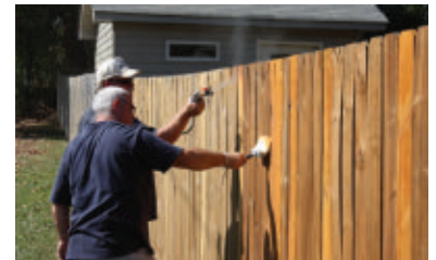
A two-man spraying-and-brushing crew can speed up completion.
