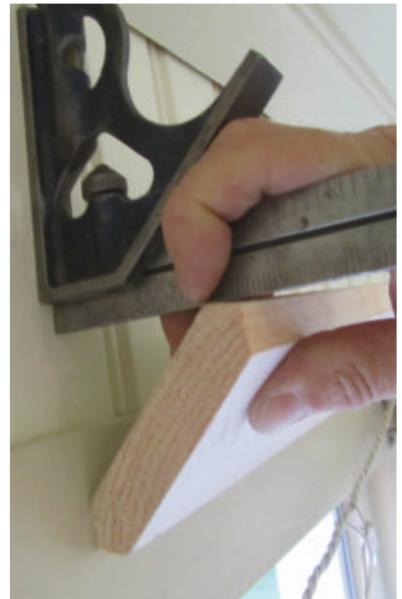
A scrap block was used to guide the layout.
