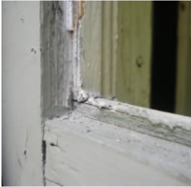
The bottom and sides of the window are built with a rabbet to house the glass pane.
