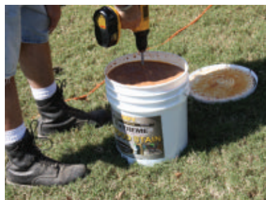
Always thoroughly mix the stain to evenly blend the solids and ensure a consistent color tone throughout the project.
