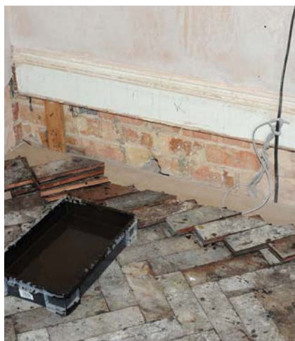
Fixing some existing skirting boards
