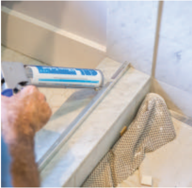
The U-channel is screwed to curbing and then sealed with silicone.
