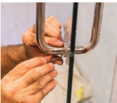
Finally, the installer tightens the shower door handle.
