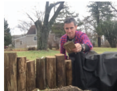
Install the semi-circular wedges with 3-inch screws. I started the screws first to make it easier.
