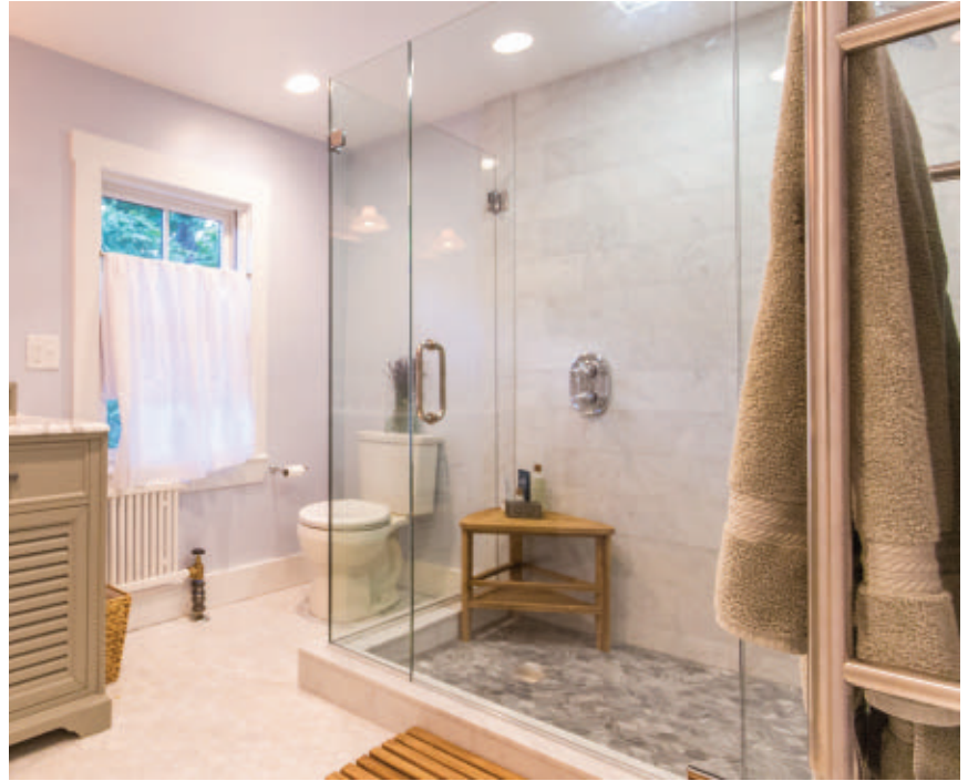
After: Shower glass enclosure system installed.
