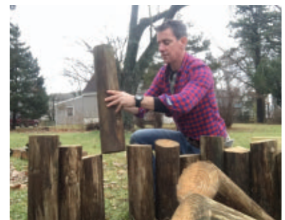
Mix and match the last few poles to get a combination that works. Note that the space on the left of the photo is for the hose chase. I kept it open by leaving a pole loose.
