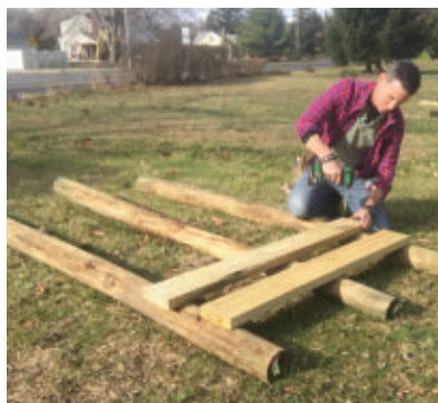
Build a sawbuck to stabilize the work.
