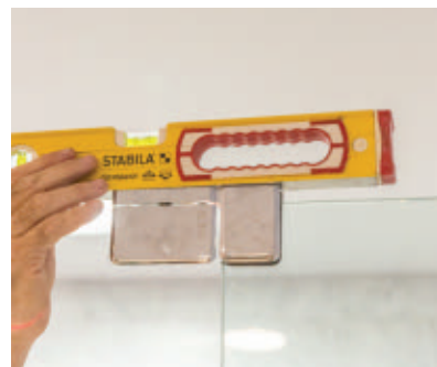
The door and hinge are aligned with the adjacent fixed glass panel.
