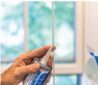
Silicone is applied to all interior edges of glass and U-channel.
