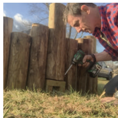
Fasten the last pole on top of the hose chase. Toe-screws into the chase locks it together nicely.
