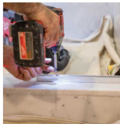
The U-channel installs with #8 1-1/2" SS screws and anchors.
