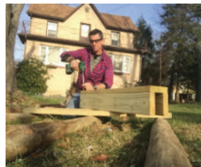
Make a U-shaped channel for the hose to run through.
