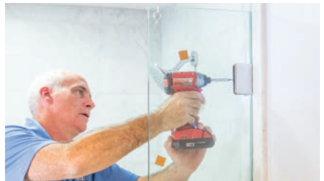
The stationary glass panel is secured to the wall.
