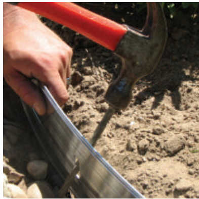
Hammer the stakes at 45 degrees.
