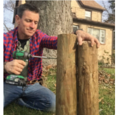
Rock 'em and lock 'em. Make sure the posts are reasonably plumb first.
