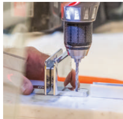
The shower curb is pre-drilled for the shower door pivot hinge.
