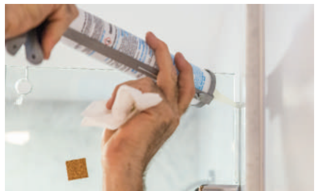
Silicone is applied to the vertical glass panel.
