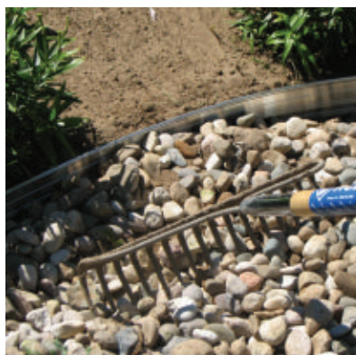
Backfill 1/2" below the edging.
