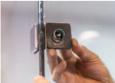
These 90-degree brackets secure the fixed glass panels together.
