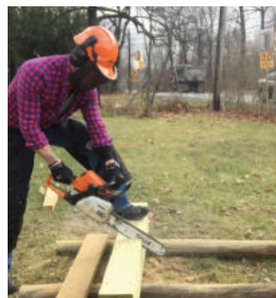
Cut the chase to length. Be careful of fasteners.
