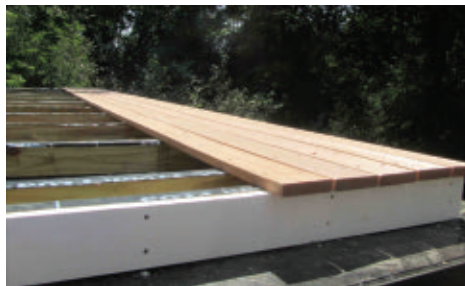
After sheathing and trim boards were installed, the deck boards came next.
