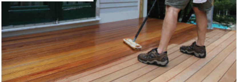
Before completing the rail system, exterior wood stain was applied while the crew had unobstructed access to the decking.
