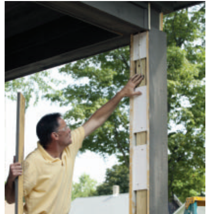
Dry-fit the column-wrap components to make sure no further adjustments are necessary.
