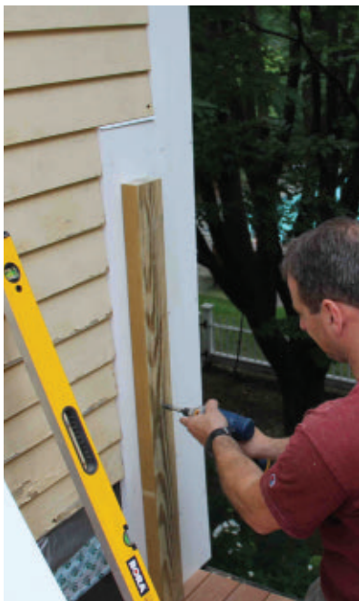
A 2x4 was used as the framing for the half post sleeve.
