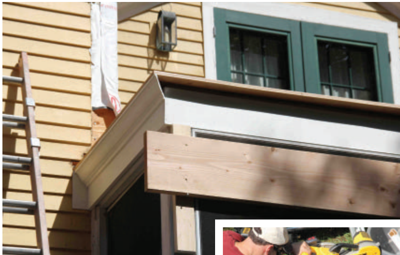
New PVC fascia and crown molding were installed for a decorative enhancement.
