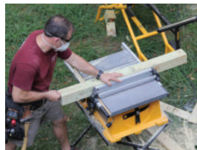
Some of the width had to be ripped off the 4x4 posts so they fit into the post sleeve supports.
