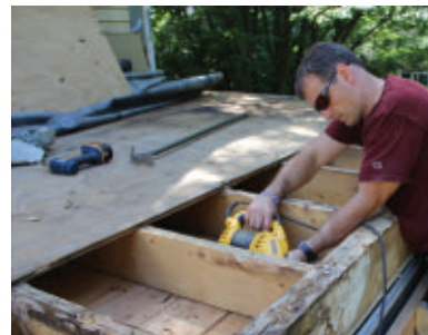
The rotted wood was cut away from the framing.
