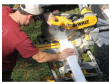
The PVC post sleeves were trimmed to height on a miter saw.
