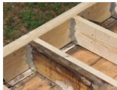
New joists were "sistered" alongside the original framing members and supported on the ends with metal hangers.
