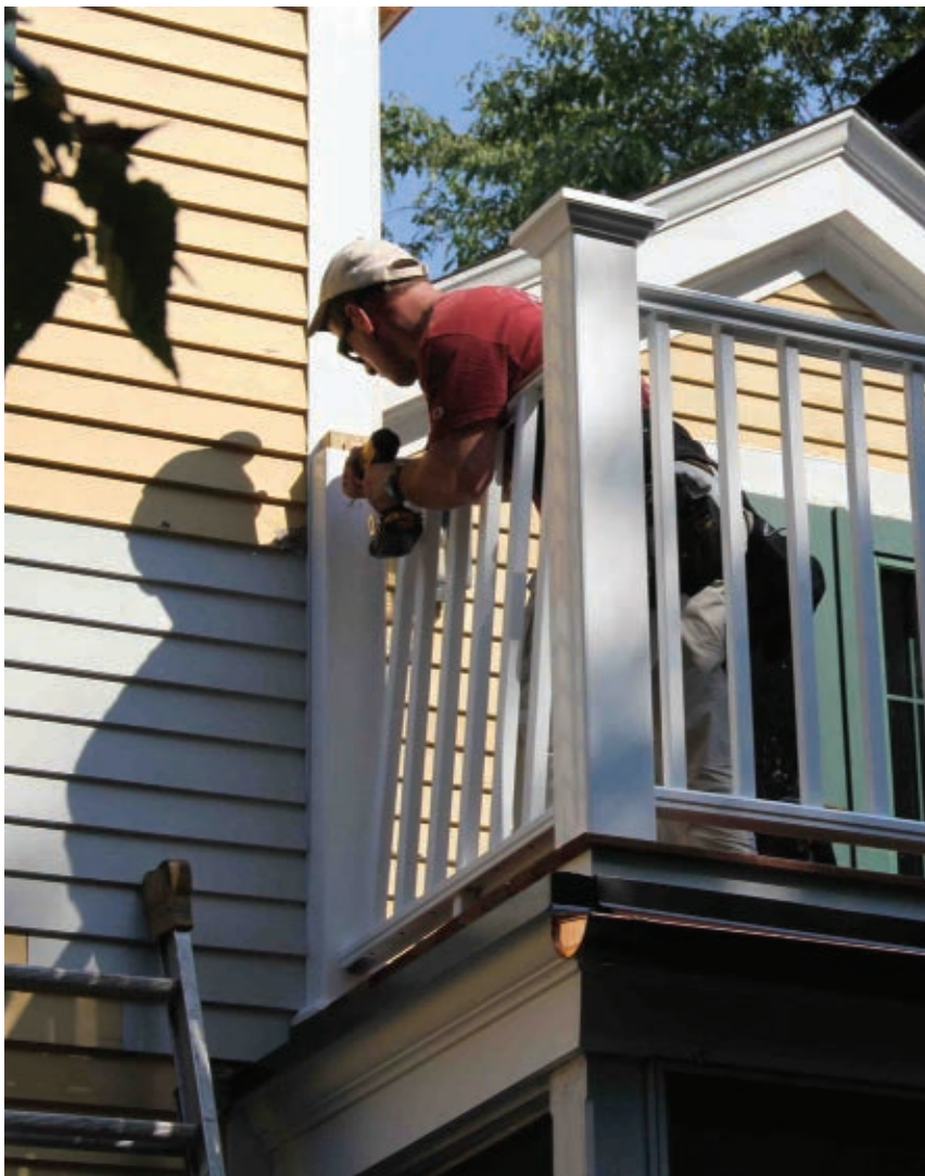
The final rail section tied into the area of siding that required replacement.
