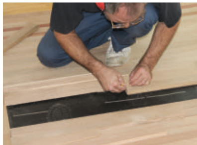
Where the field rows terminate into the exposed tongue of the border, carefully mark the length of the final boards.
