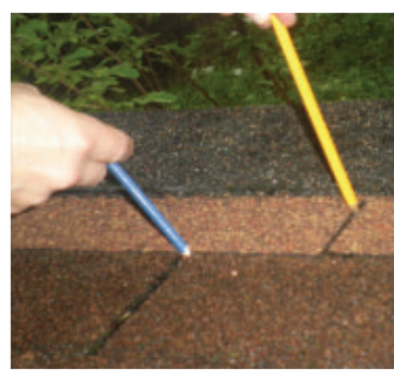
Stagger all of the tabs to keep water out of the roof system.
