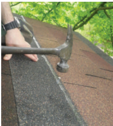
Nail the new shingles down.
