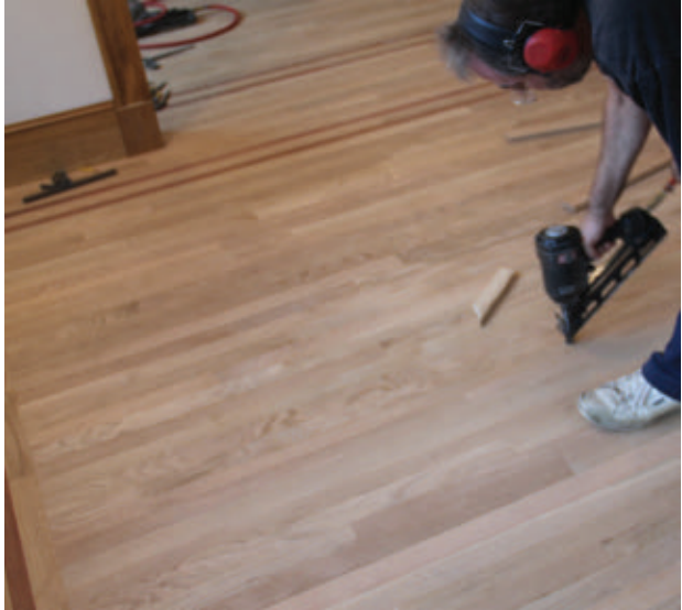
Face-nail to fasten the final row securely.
