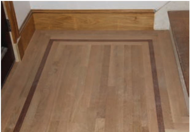
One rule of thumb is to use a single feature strip in smaller areas and double strips in actual rooms or larger spaces.
