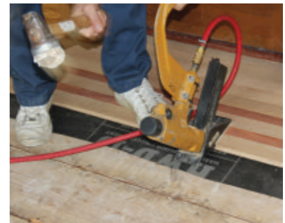
The flooring was fastened over a moisture barrier using a heavy-duty flooring stapler.
