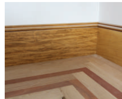
The ends of the intersecting rows of the border use a consistent and overlapping pattern in the corners, not unlike a herringbone pattern.
