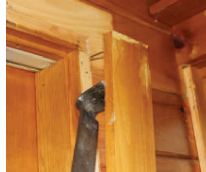
The first step to remove the windows was to pry away the interior trim.
