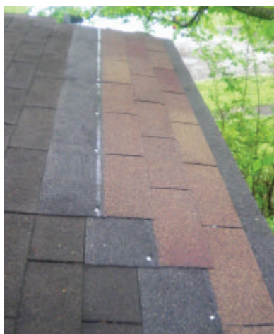
Shown are the first three courses of new shingles laid over the old shingles.
