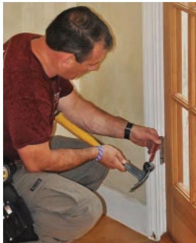
Always remove the lower hinge pins first and work your way to the top.
