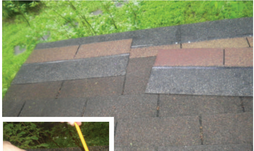
Stagger all of the tabs to keep water out of the roof system.
