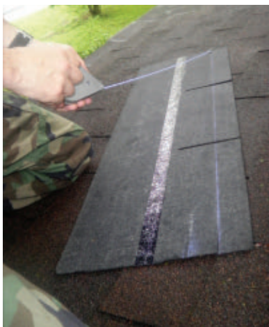
Use a chalk line to mark a straight line on the back side of any shingles that need to be cut.
