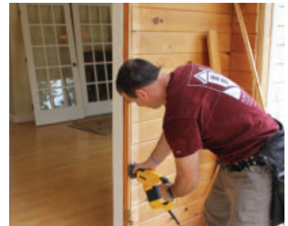
Cut the jamb fasteners with a recip saw.
