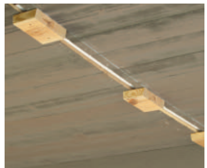
Steve Roth installs nailing blocks that slip inside the hollow beams.
