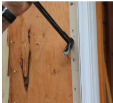
Extract each of the nails from the flange to free the window.
