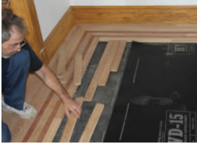
Stagger the joints of floor boards at least 4 to 6" between adjacent rows.
