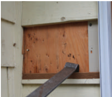
The siding was pulled off to reveal the window's nailing flange.
