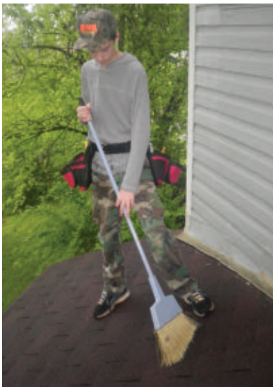
Sweep off the old roof before starting work so it is free of debris.
