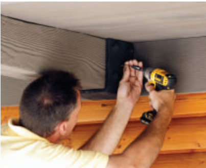
The beam straps were installed as a finishing touch.
