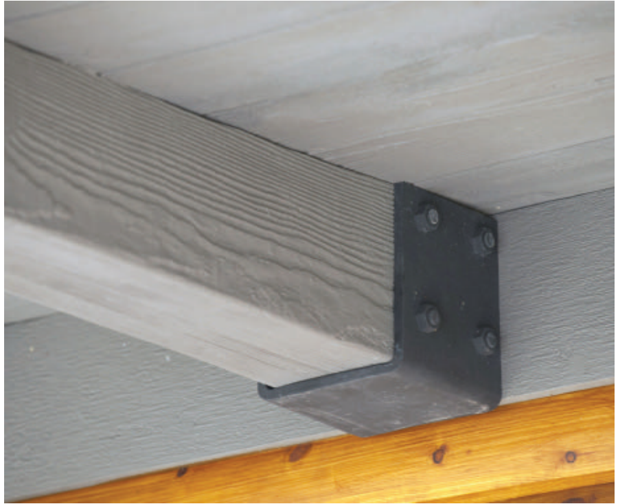
The beam straps were installed as a finishing touch.
