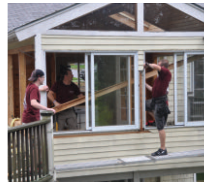
Some of the upper-level windows required careful staging for removal.
