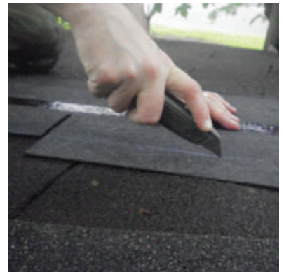
The easiest way to cut shingles is to cut them on the back side with a utility knife.
