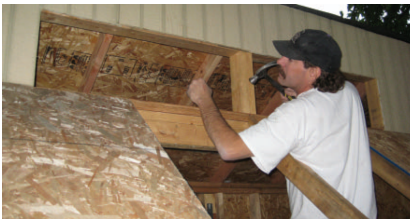
The clerestory required some adjustments.
