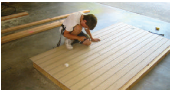
The author's son gets into the act applying T1-11 siding to the front wall section.
