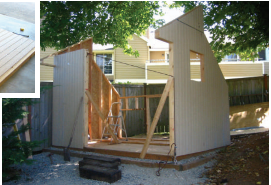
The author's son gets into the act applying T1-11 siding to the front wall section.
