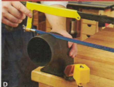
D Clamp the flange of the elbow to your workbench to steady it. Then hacksaw off the straight portion of the unflanged end.
