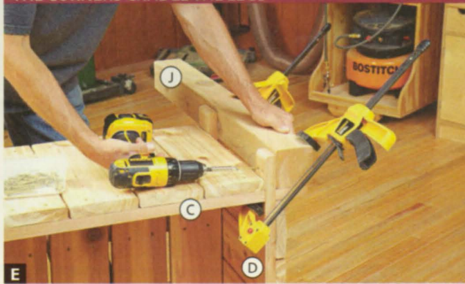
E After drilling and countersinking the pilot holes, apply glue to the faces of the rails (A–D) and screw the legs (J) in place.
