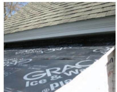
The roof sheathing was protected by Ice & Water Shield.
