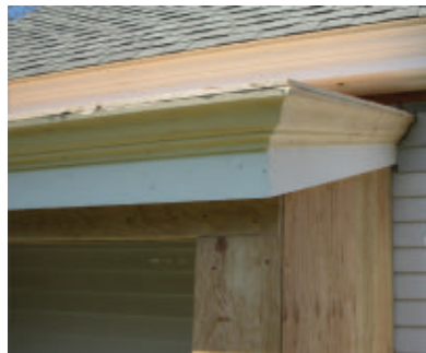
The crown molding provided a nice finish detail.
