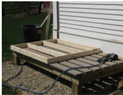
The walls were assembled and tilted into place.
