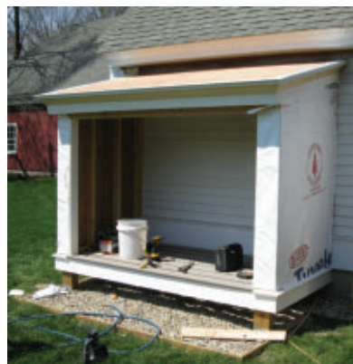
The sheathing was wrapped in building paper.
