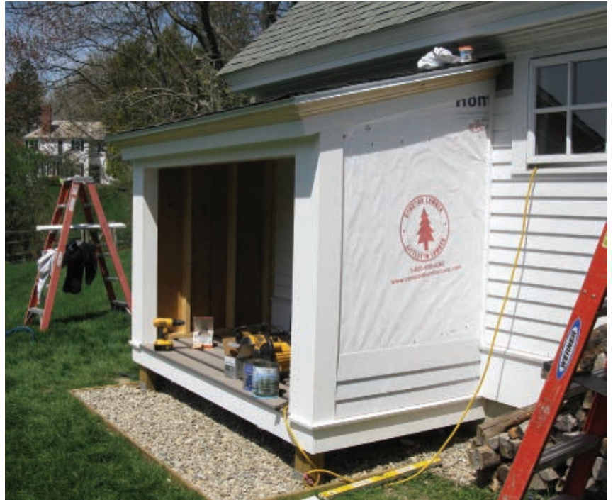
The walls were then sided with pre-primed Western Red Cedar clapboard.
