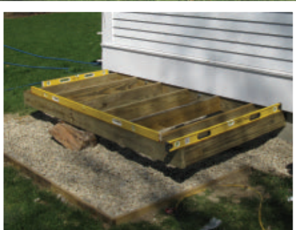
A gravel-covered base lined the foundation.
