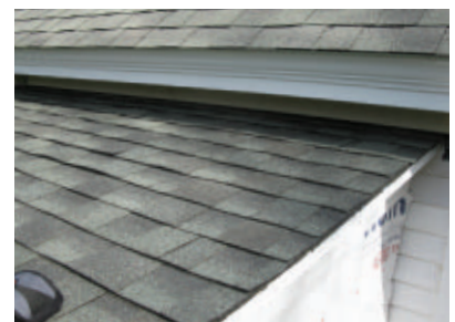
The new roofing shingles matched the existing house roof.
