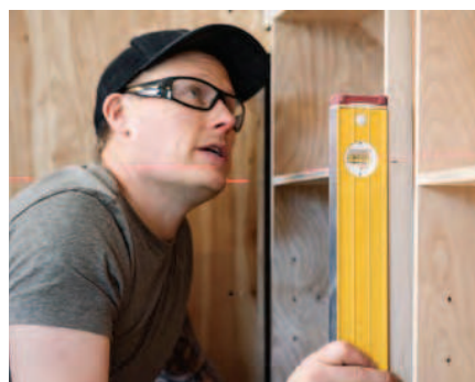
Laser level and plumb. Set to the height of the cabinet's fixed shelves, a laser line is used to ensure each carcass is at a level height with the adjacent units. Young uses a level to check that each unit is installed plumb.
