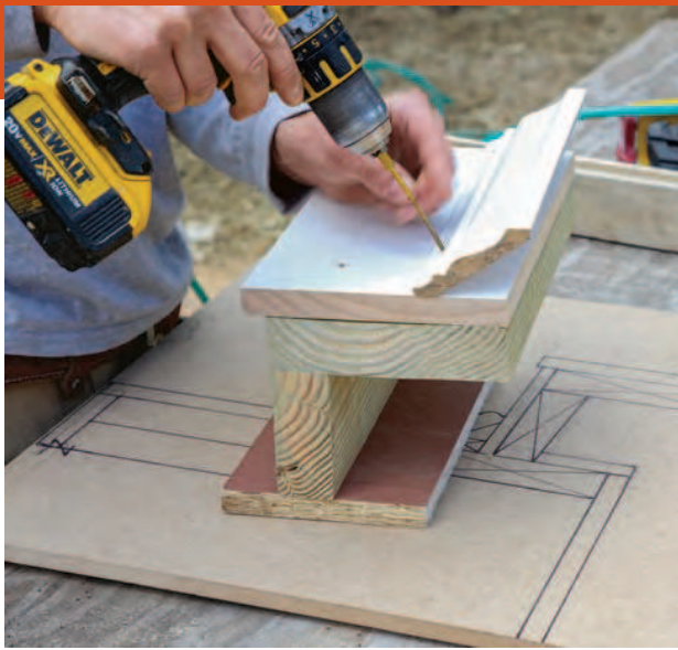
Make a mockup. Using a full-scale cross-section drawing as a template, build a mockup of the bare-bones cornice assembly, being sure to include enough of the trim to get an idea of how the new will tie into the old.
