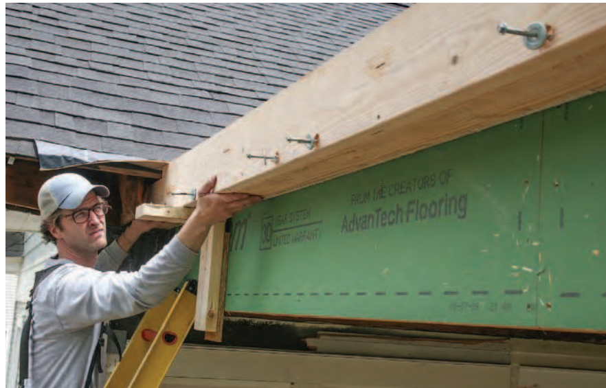
A clever corona. After cutting, assembling, and waterproofing the gutter trough, set it atop temporary brackets aligned to the datum line, freeing your hands for final positioning and stress-free fastening.
