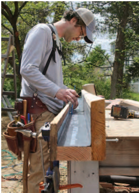
A clever corona. After cutting, assembling, and waterproofing the gutter trough, set it atop temporary brackets aligned to the datum line, freeing your hands for final positioning and stress-free fastening.
