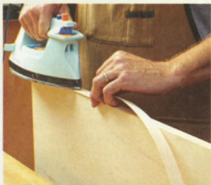
Using a dry iron set on medium heat, press a slightly over-length strip of edging onto the plywood. Position the edging by feel ahead of the iron, maintaining an overlap on both sides.
