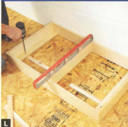
L Use shims to level the ladder base in both directions. Once level, attach the base to the floor, screwing through both cleats and shims.
