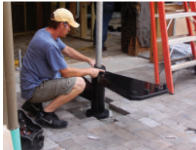
The treads and spacers slide over the pole.
