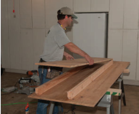
Place the main table surface on the 2x4 runners.
