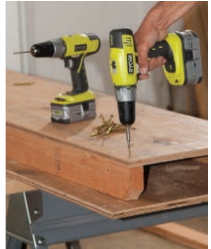
Pre-drill and screw the plywood to the runners with drywall screws.
