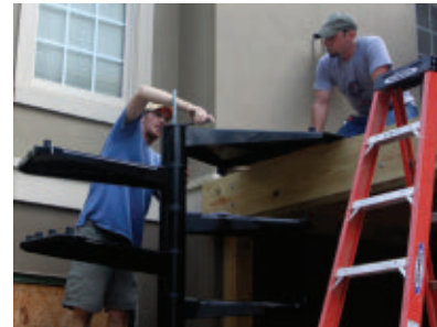
The staircase shown has a mezzanine landing.
