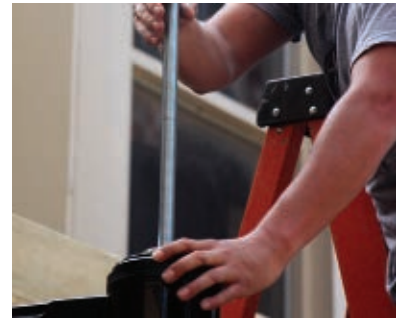
Add the second section of the pole and continue assembling the treads.
