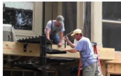
The next step is baluster installation.
