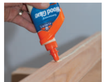
Apply wood glue to the non-chamfered edge of the 2x4s.
