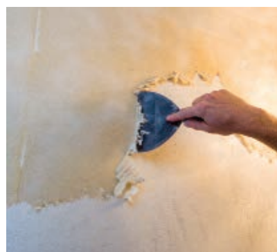
A joint knife or wide putty knife make good tools for scraping off the wet wallpaper backing.
