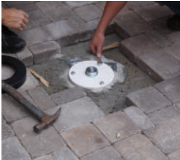
Install the base plate.
