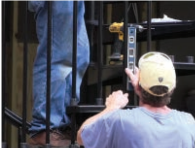
Keep the balusters plumb when assembling.
