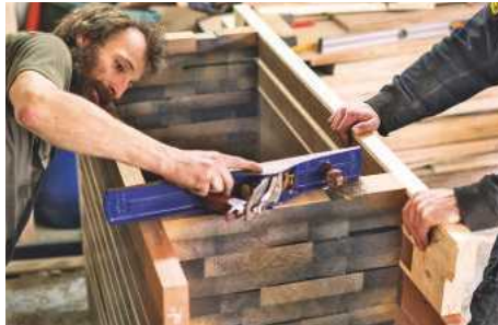
Jack Badger leads the way in preparing the frame sections and keeps a careful eye on quality control
