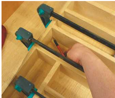
▲ Pic.12 Mark out all intersections ready for the biscuit slots to be cut
