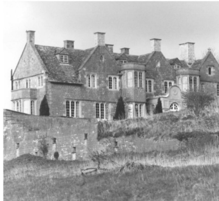
Hilles House: stone slate replaces the original thatch lost in a fire
