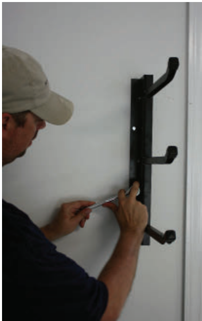
The Racor 450 Rack comes with heavy-duty lag screws that must be mounted to stud framing.
