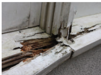
On some windows water intrusion had resulted in sills that were completely ruined by rot.
