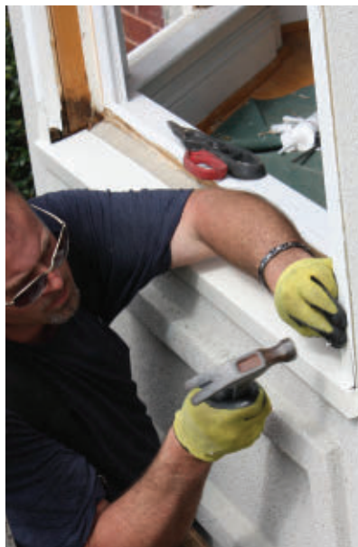
The sill wrap is the first piece to be installed so the window can be placed over it.
