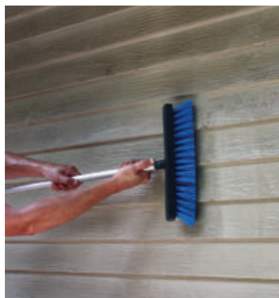
Many house and siding cleaners claim to work without scrubbing—but we scrub anyway.
