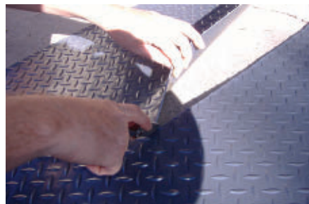
If necessary, trim the covering with a utility knife or scissors.
