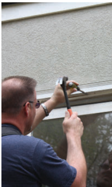
Stop molding surrounds the top and sides of the windows.
