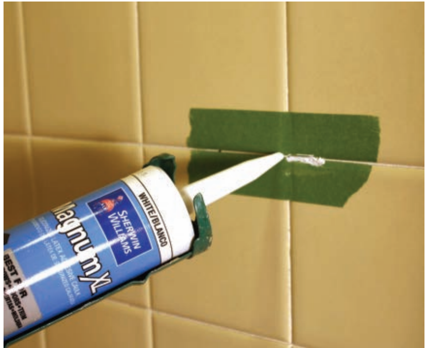
Waterproof caulk can be used to fill small cracks in tile grout.
