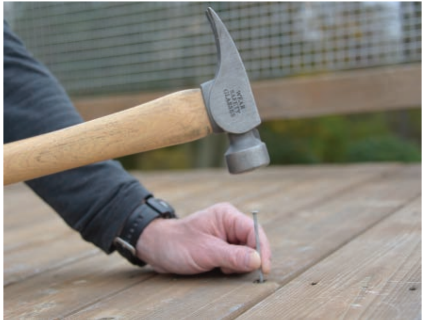
Replace loose fasteners with quality decking screws or spiral/rink-shank nails. Also, inspect the framing connections beneath the deck.
