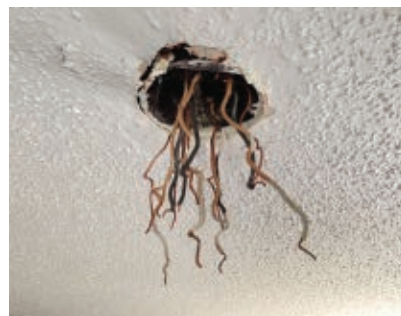
It's a good idea to label your wires for reconnection, because once you remove all the wire nuts, you may have a tangle of wires like this to sort through.
