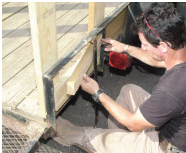
Add blocking as needed to create a wall around the trailer's angle iron projections.
