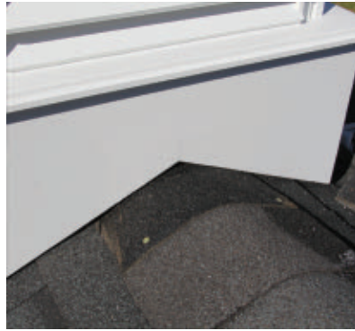
Use the ridge shingles that you removed, if in good condition, to make any necessary patches or to cover any roofing you removed.
