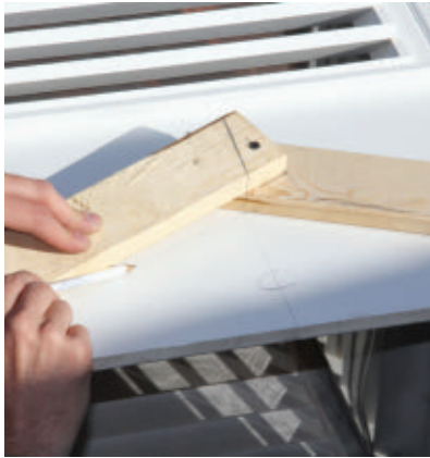
Scribe the roof pitch onto the cupola. Cut the angle with a jigsaw.
