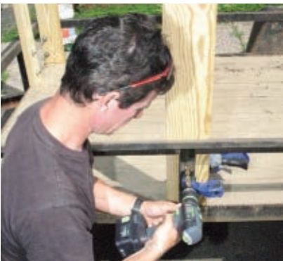
Clamp the stave square to the trailer frame and drill the hole for the through-bolt.
