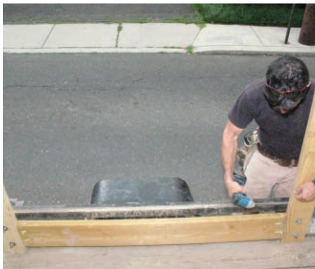
I span the trailer's wheel well with blocking on the inside of the trailer, installing the boards flush with the staves.
