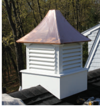
Bring the cupola to the roof and test the fit.
