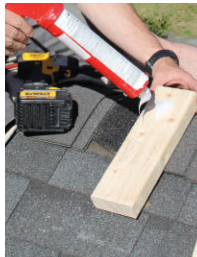
Pre-drill holes in the 2x4 mounting blocks and apply silicone to the bottom of the prior to attaching them to your roofing.
