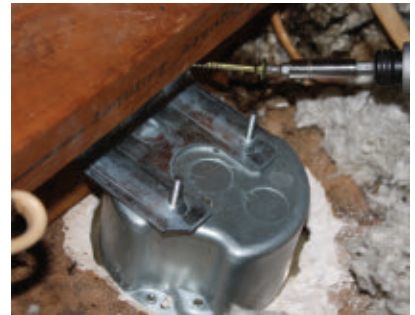
In my situation, I attached the fan box to the side of the joist using heavy-duty R4 screws from GRK fasteners.
