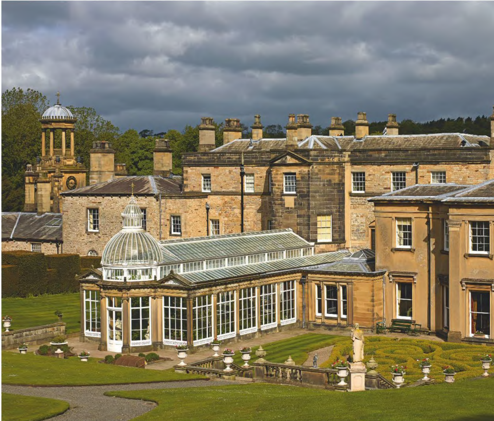
Fig 7 above: The back of the house is built into the hill. Its conservatory, built by Andrews and Delaunay of Bradford after 1838, and drawing rooms overlook a formal garden by W. E. Nesfield
