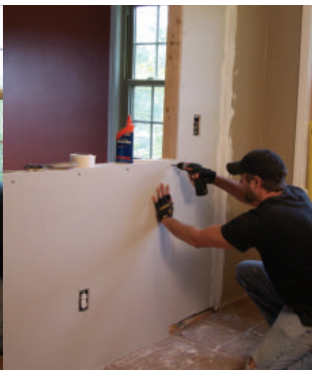
The jack studs were notched to accept the countertop.
