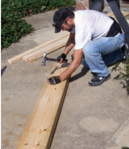
The header was built from 2x10's and plywood.
