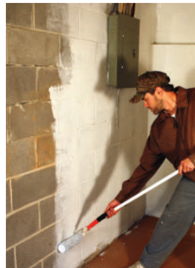
Roll on the masonry waterproofer in 3' sections and then back-brush it into the block.
