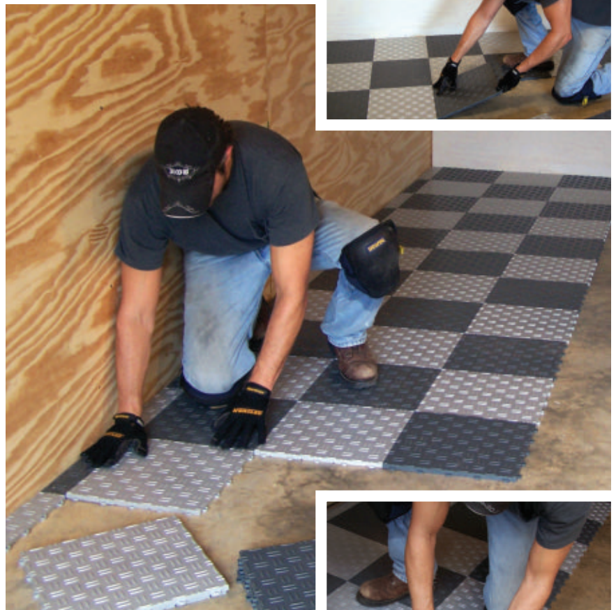
Install rows 4 through 6 along the adjacent wall toward the garage door.
