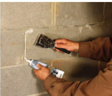
Scrub away any loose debris and fill cracks and holes with concrete patch.
