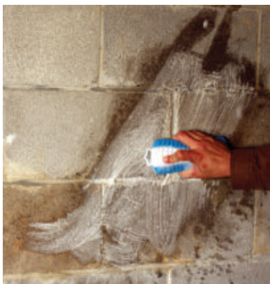
Scrub away any loose debris and fill cracks and holes with concrete patch.
