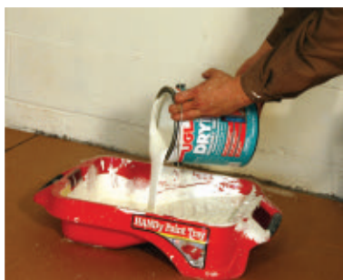
A thick-bodied product like Drylok fills the porous masonry surface to prevent seepage.
