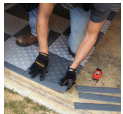
Install beveled edging at the end of the floor, staying clear of the garage door.
