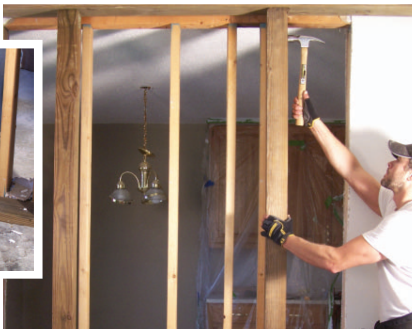
Load-bearing walls require temporary support walls to carry the weight of the overhead structure.
