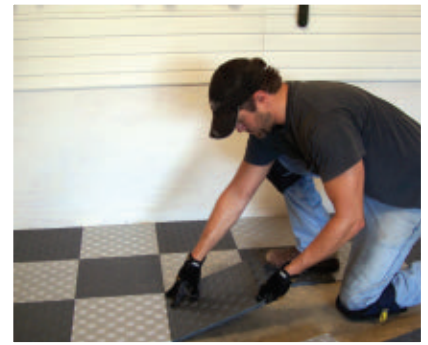
The tiles snap together easily along the edges.
