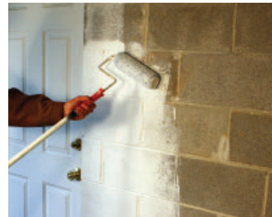
Roll on the masonry waterproofer in 3' sections and then back-brush it into the block.
