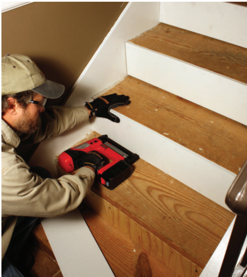
The risers are fastened with construction adhesive and finish nails.
