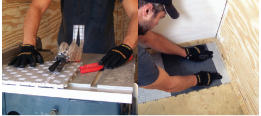
Tiles can be cut with a table saw, circular saw or jigsaw.
