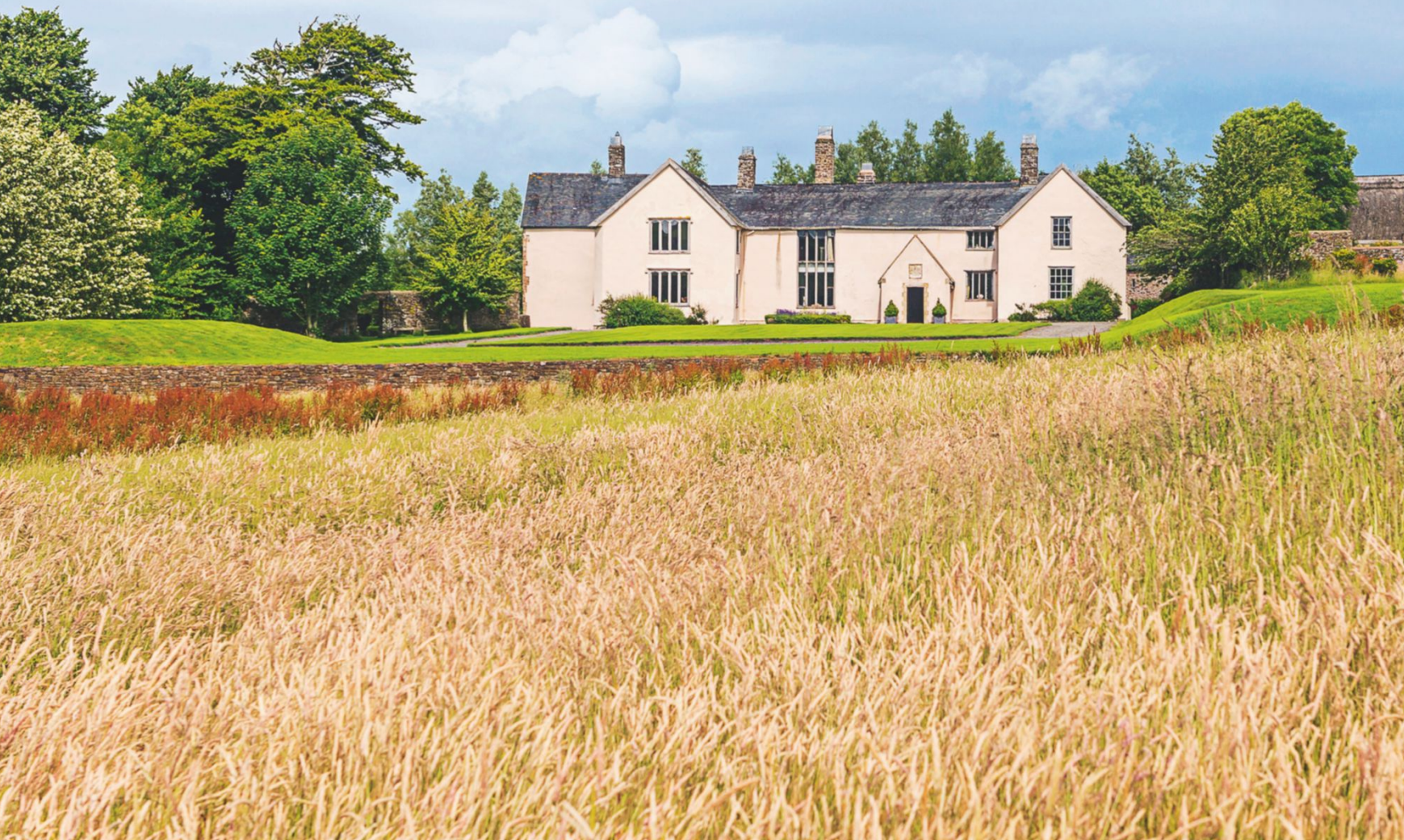
Fig 1 preceding pages: The parlour. Fig 2 above: The house in its landscape. The central hall is entered through a modern porch and the cross-wing to the left contains the parlour and great chamber. That to the right was rebuilt in the 19th century
