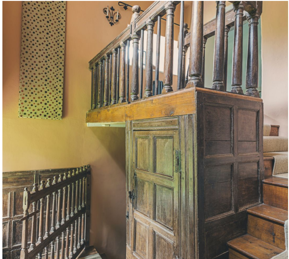
Fig 5: The dog gate on the 17th-century principal stairs. The four flights are arranged around a panelled core, a form that had become unfashionable by the 1630s
