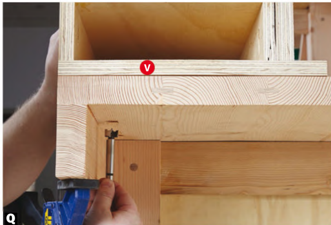
Q Mark the dog holes. Push a \frac{3}{4} " Forstner bit through two dogholes under each wing and the saw mount. Give the bit a tap to mark the centerpoint of each doghole.
