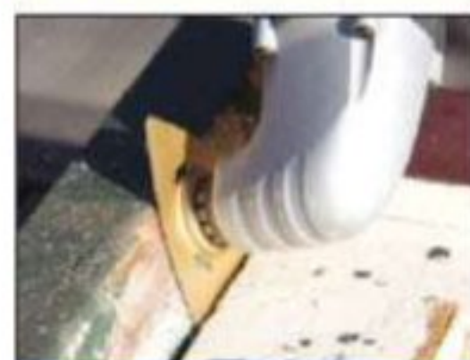
AGGRESSIVE PAINT REMOVAL
