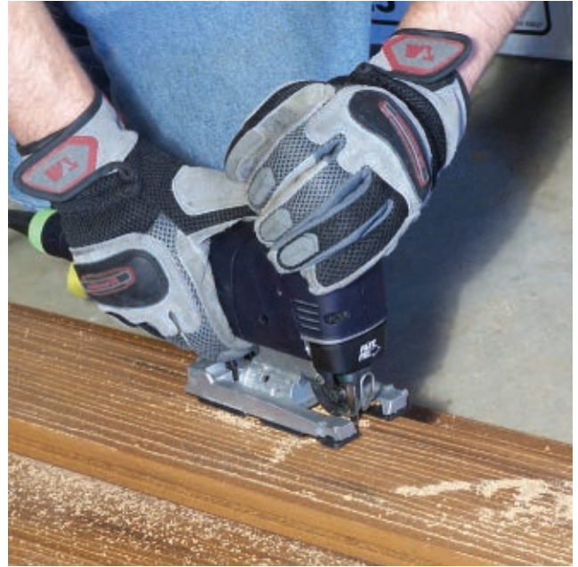
On the "house" side of the deck, a few boards had to be ripped to width, and one board had to be notched to fit around a chimney.
