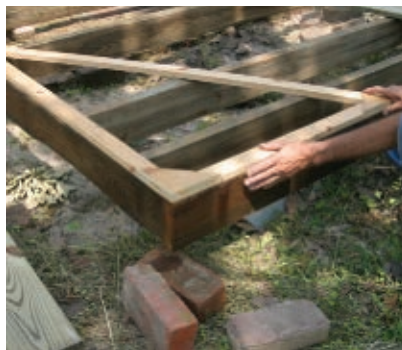
A large, shop-made 90-degree triangle makes it easy to square up the deck.
