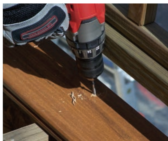
The first new composite board was installed flush with the outside edge of the deck. The first board was fastened to the framing with square-drive composite decking screws.
