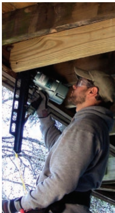
A pneumatic framing nailer is a great help when fastening the joists.
