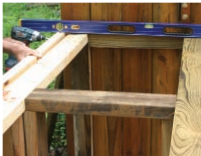
The concrete top is formed in place. Form boards are anchored to the cabinet framing.
