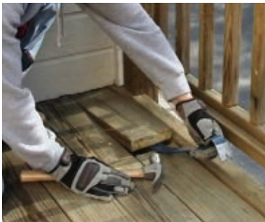
Once it was cut, the board pulled up easily with a small pry bar.
