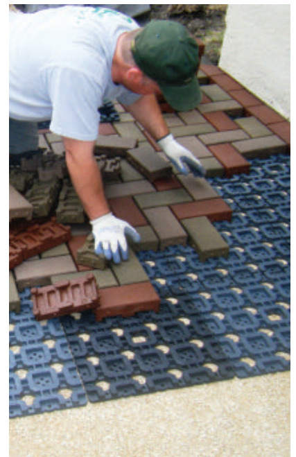
AZEK pavers weigh much less than concrete and install on a grid.
