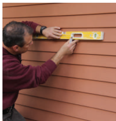
On the outside of the wall, use a level to connect the four corners of the door tunnel.
