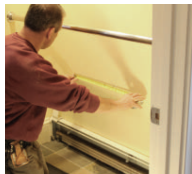
Carefully lay out the pet door location square to the floor.
