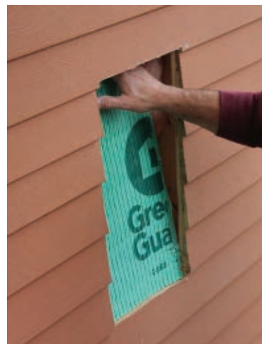
Remove the siding and plywood sheathing from the tunnel.
