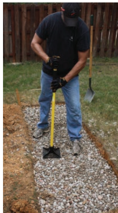
Add a gravel base for the slab.
