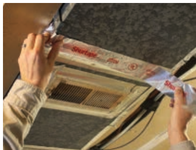
Use foil tape for an airtight seal around ductwork.
