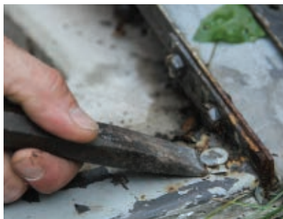
The old fasteners were pulled out of the concrete foundation.
