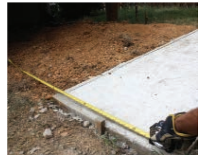
After the concrete fully cures, it's ready for use as a walkway or footing.
