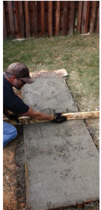
Screed the concrete even with the form.
