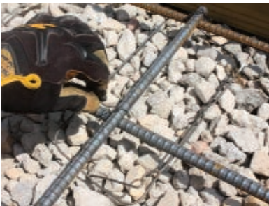
Secure the rebar grid with wire ties.
