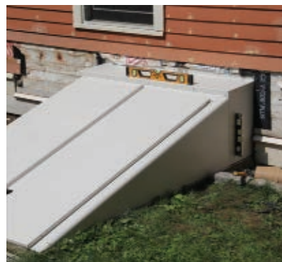
Level the door carefully and fasten according to the instructions.
