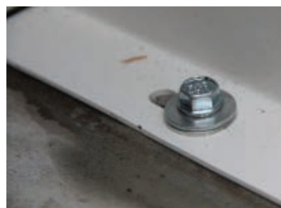
For extra holding power, the fasteners for this project were upgraded from the recommended concrete screws to wedge bolts and expansion bolts.
