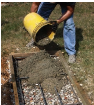
Apply the concrete. I mixed it one bag at a time but should've rented a mixer.
