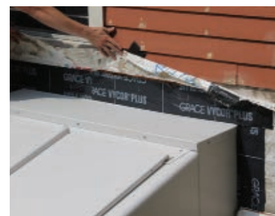
The flange of the door was sealed with rubber flashing.
