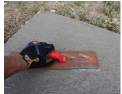
Float the surface of the slab to bring the cream to the top.
