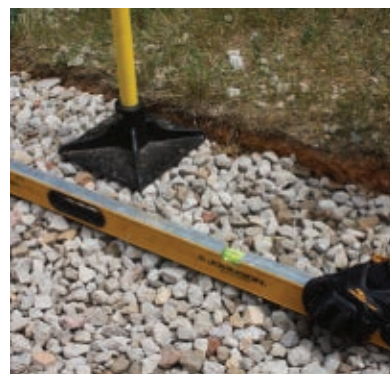
Tamp down and level the gravel bed.
