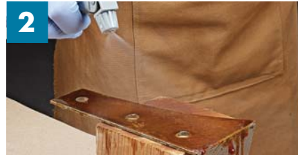
2 Add Solution. The solution starts working as soon as you spray it on. Flood the surface, then let it sit overnight.
