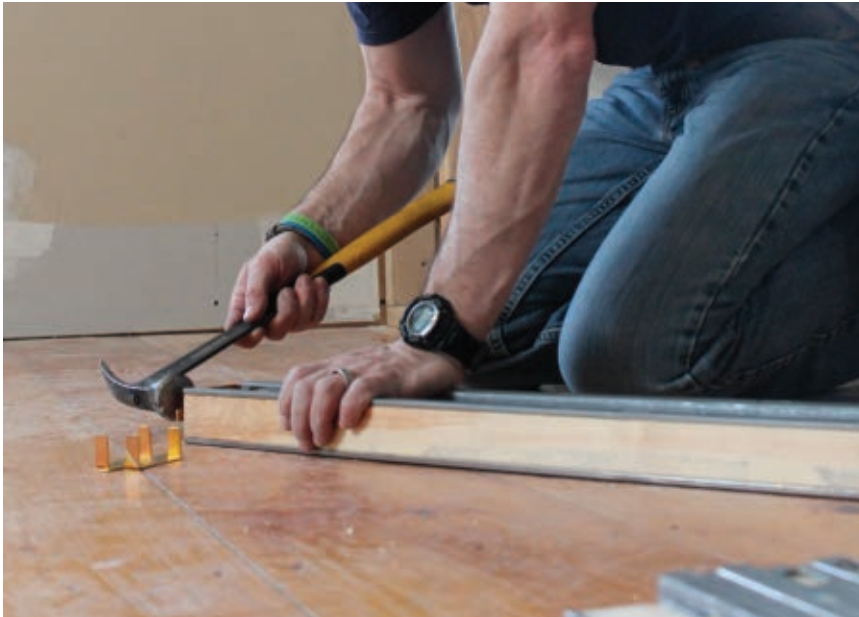
Clips hold the stud assemblies together. Tap them on with a hammer and make sure to orient both studs the same way so the nailing slots face the back of the drywall.
