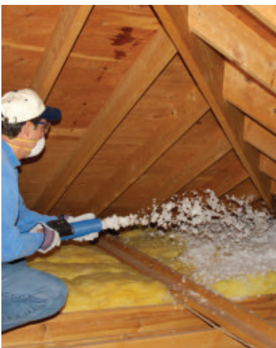
Some types of insulation can be blown into the attic using a machine that many home centers offer free of charge. (photo courtesy Certainteed)
