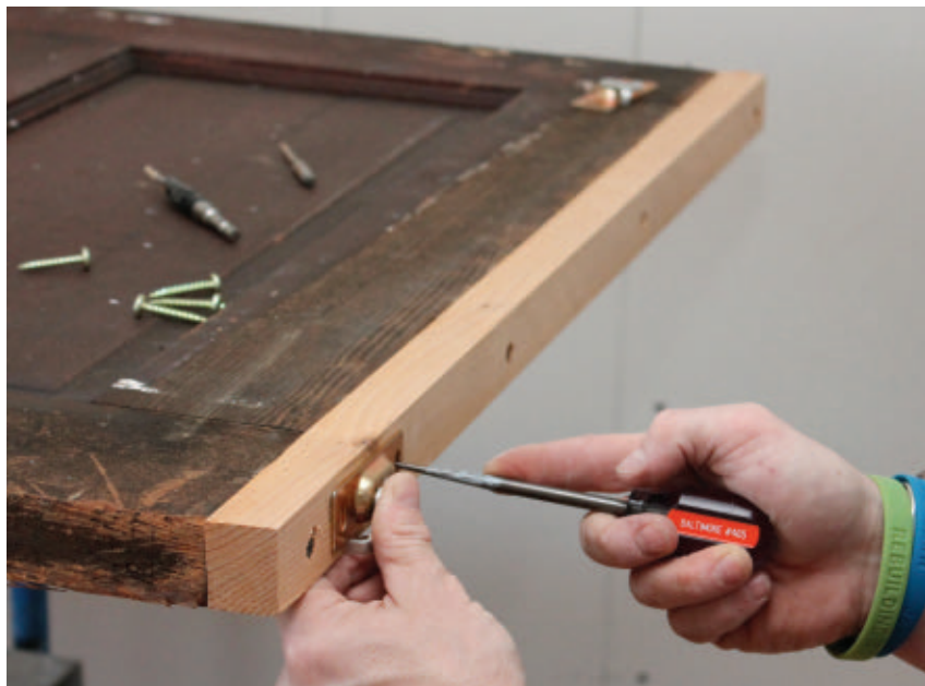
The only difference between our installation and a typical installation is that we added a header strip to our vintage door. The end grain had taken a beating over its one hundred years of service (and 30-years or so of sitting in an attic with a roof leak over it).
