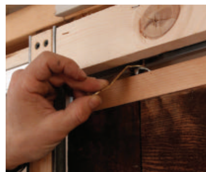
Install the stops so the doors kiss when they close. Leave your power tools out of this one, though. Just snug them up with a screwdriver. Use the world's smallest wrench to adjust the doors into plumb.
