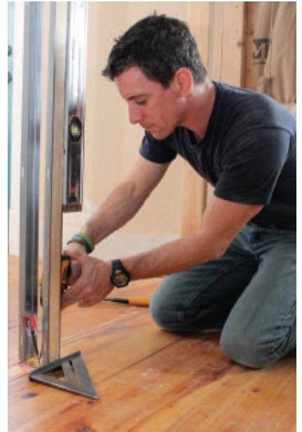
Installing the stud assemblies on the layout marks is tricky because everything is loose and wobbling around, so I use a few tricks to keep them honest. To help keep them right on the line, I drive my awl into one of the screw holes while I pilot and drive the other screw. And, I hold a layout square on the line so I can tell if the stud moves.
