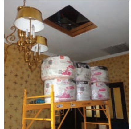
Set up a work station that facilitates moving materials into the attic.
