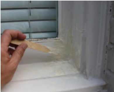
The PL FIX product can be cut and shaped to match existing wood profiles.
