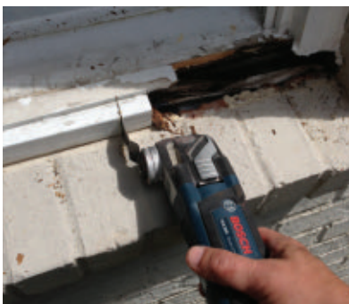
An oscillating multi-tool like this Bosch Multi-X is a great gadget for cutting out damaged wood.
