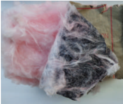
The paper facing of fiberglass insulation contains a plastic layer that serves as a moisture barrier to the attic space.
