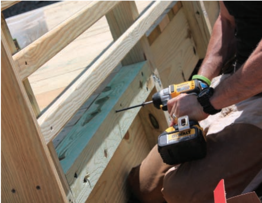
Forget nails or deck screws, we impact-drove 6" LedgerLOKs into our 4x4. Bam!
