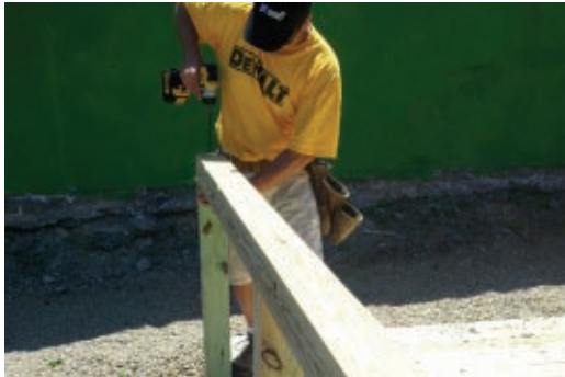
We fastened a 4x4 top cap to our 4x4 posts for a beefy, linear look.
