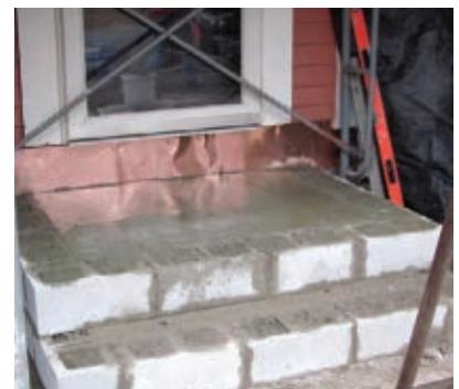
Concrete block prior to stone installation
