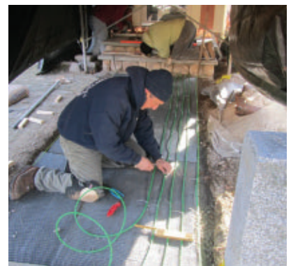
Laying out walkway cables
