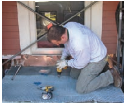
Install tapcons into mesh
