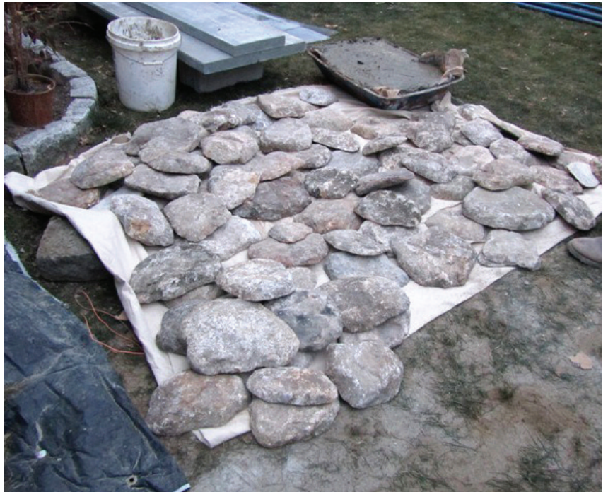
Veneer stones for the step risers
