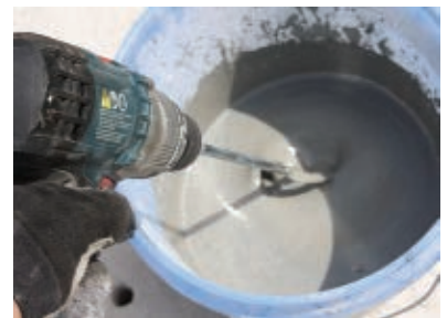
A drill and paddle blended the agent into a smooth slurry.
