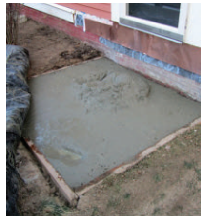
Concrete pad for stoop
