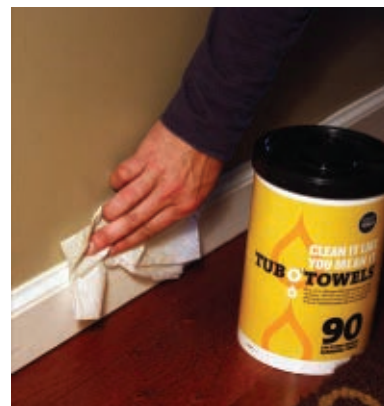
Clean the work area thoroughly to keep the caulk clean and ensure the best adhesion.
