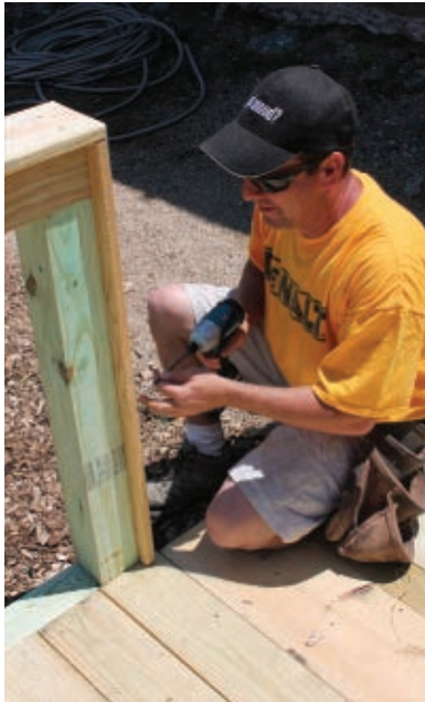
We wrapped the 4x4 rail and end-posts with 5/4 and fastened with screws.
