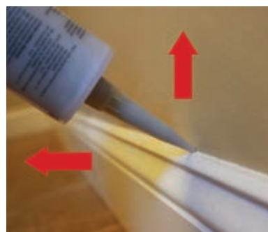
Rest the nozzle tip evenly on both sides of the joint.
