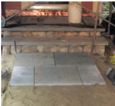
Installing the bluestone
