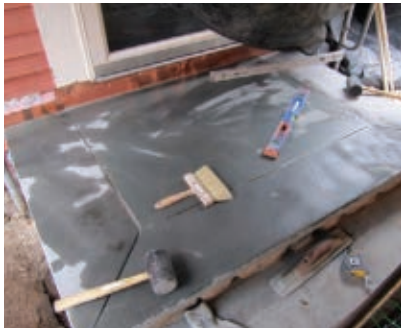
Stoop landing installation
