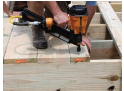
We alternated two 2x10 and two 2x6 for this deck system. It also delivers a cool look.
