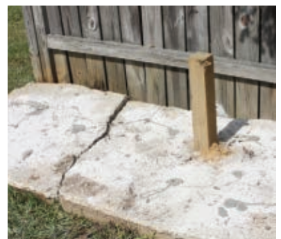
Here's the slab w/ all holes filled.
