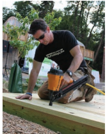
Use 3 nails per joist on 2x10. For any gun-nail decking we recommend ring-shank 16s.
