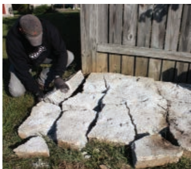
Concrete chunks ready for a wheelbarrow.
