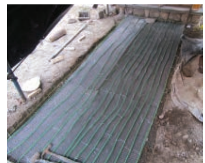
Walkway cables installed
