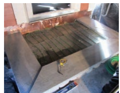
Miter cuts on the stoop
