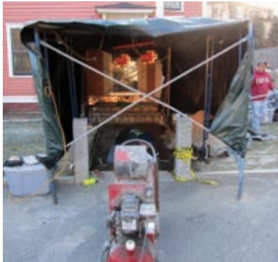
Walkway tent for heating
