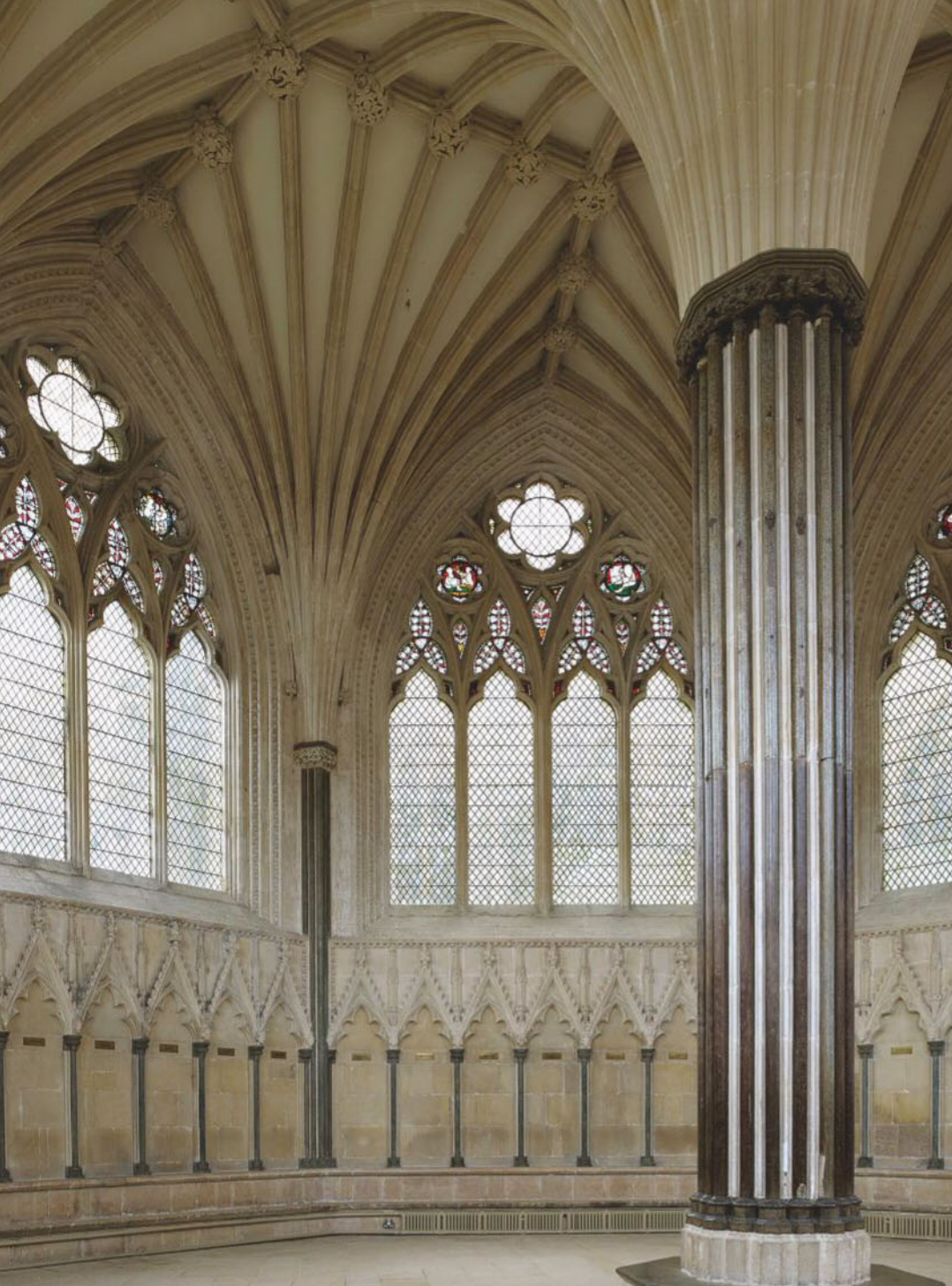
Fig 2 above: The chapterhouse interior. Its use of contrasting colours of stone accentuates the intricacy of the design. Fig 3 facing page: A stair travels from the north transept into the chapterhouse chamber. To the left, a door leads over the Chain Gate to the Vicars' Hall
