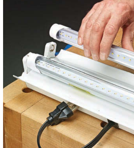
▲ Reassemble the fixture and install the new LED tubes into the tombstone sockets before reconnecting the power.
