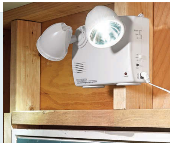
▲ Stumbling your way out of a dark shop when the power goes out can be dangerous. This fixture comes on during power outages to light the way to the door.
